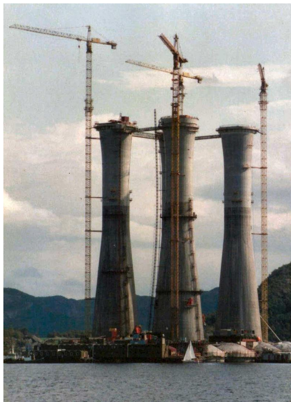
Figure 13 - Concrete Gravity Structure under construction in Norway (Wikipedia 2016)
