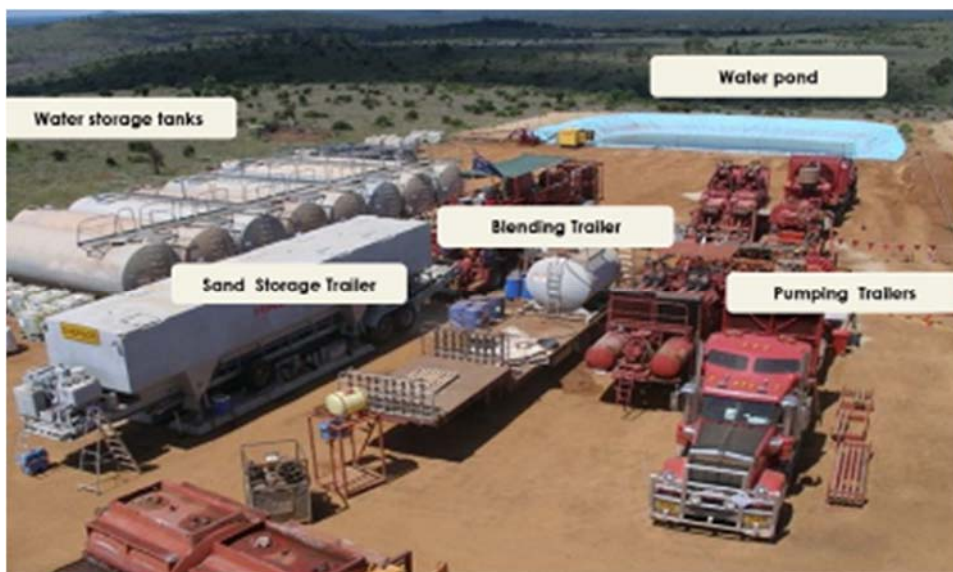
Typical On-site Hydraulic Fracturing Operation (source QGC)
